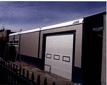
The industrial structures with insulated PVC roofs have their side walls covered with either insulated sandwich panel or insulated PVC fabric. These facilities have many uses, for example storage or workshop facilities and have also been used as production facilities.
