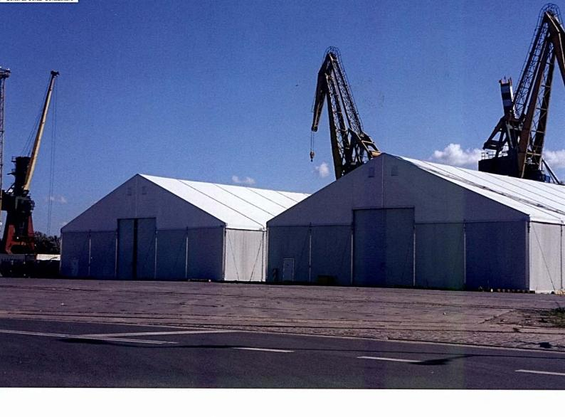
The storage structure is a semi permanent feature with a roof covering manufactured from PVC-coated polyester fabric. The covering of the side walls and end walls is available in various options: the most popular ones include PVC-coated fabric, single skin steel sheet or insulated sandwich panel.
